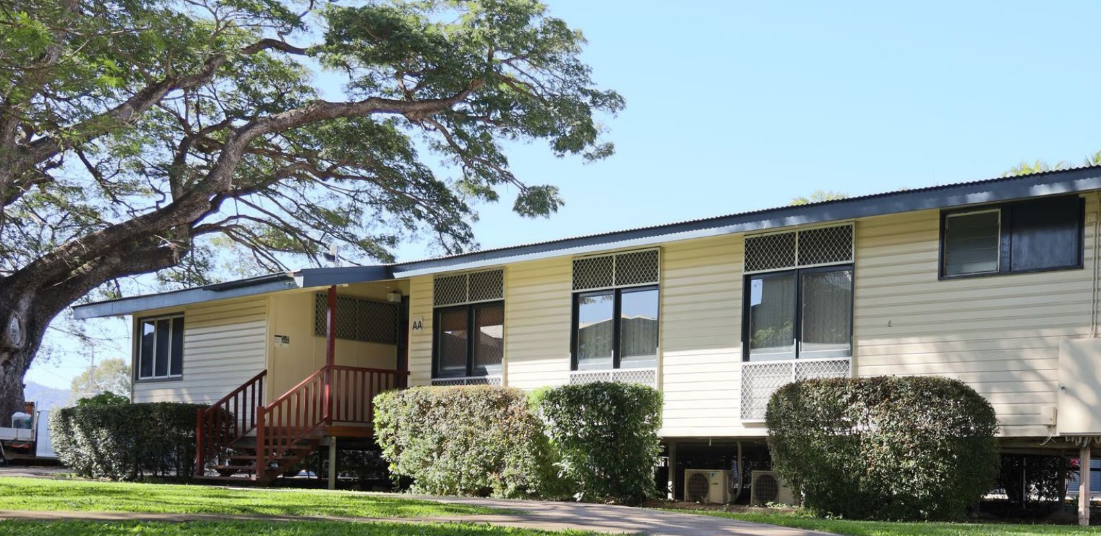
ST MARY'S EXTERIOR
